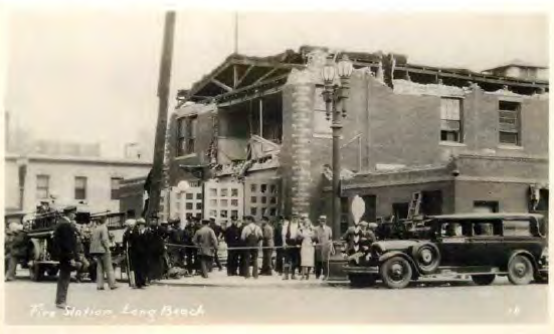
Figure 78: Fire station collapse, 1933 Long Beach (CA) earthquake. Note MFD's headquarters building dates from 1932.
