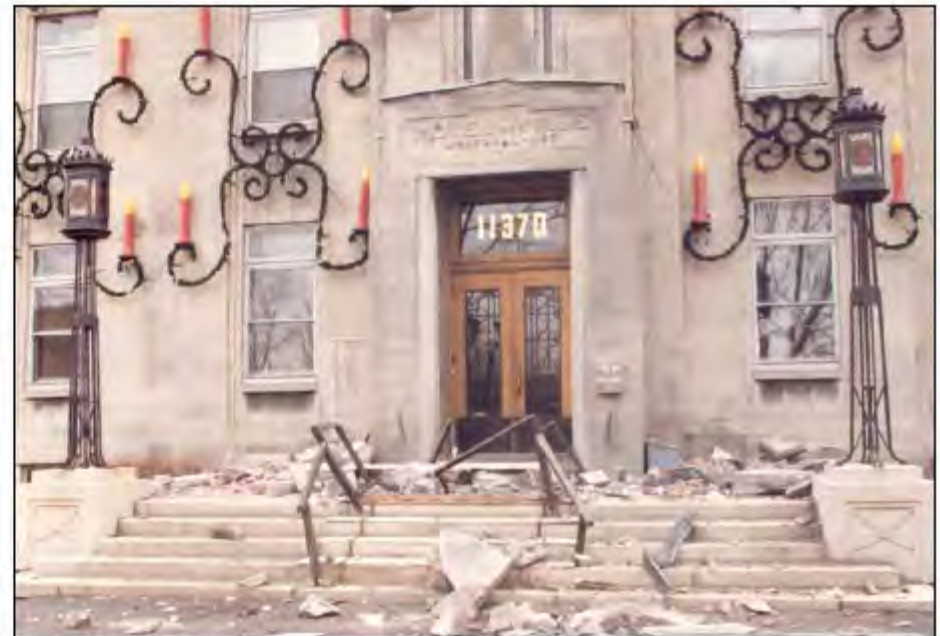
Figure 14: Loss of Montreal East City Hall masonry cladding in 1988 Saguenay earthquake.
