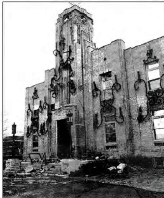
Figure 14: Loss of Montreal East City Hall masonry cladding in 1988 Saguenay earthquake.
